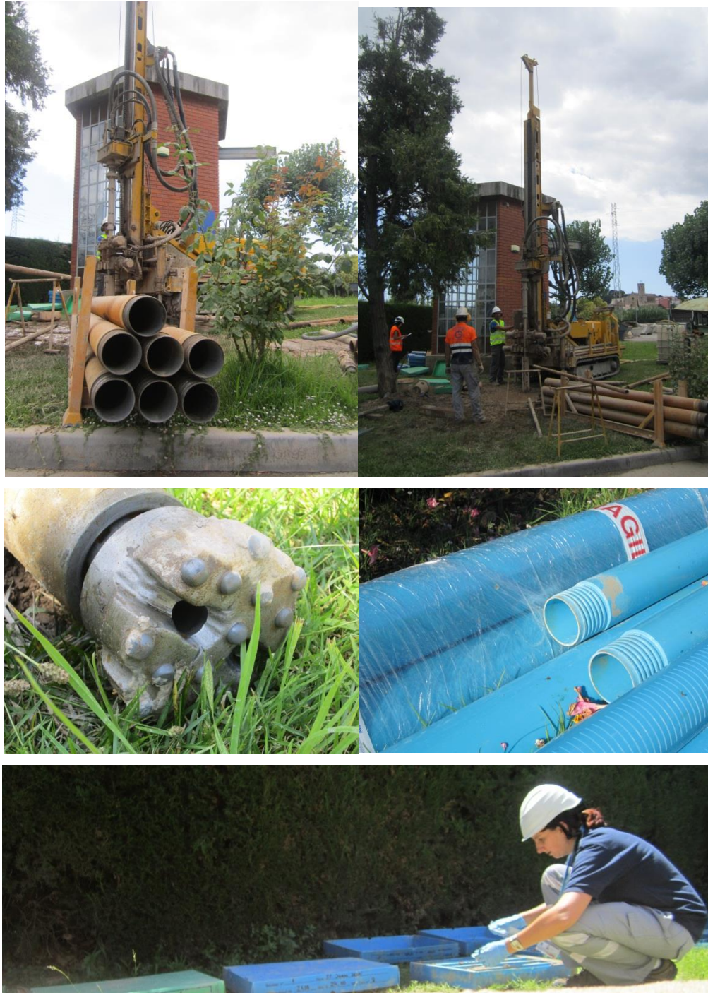
Figure 9: Drilling works of Pz1 in Sant Joan Despí
